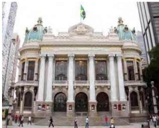
Figura 87 – Fachada Theatro Municipal RJ
